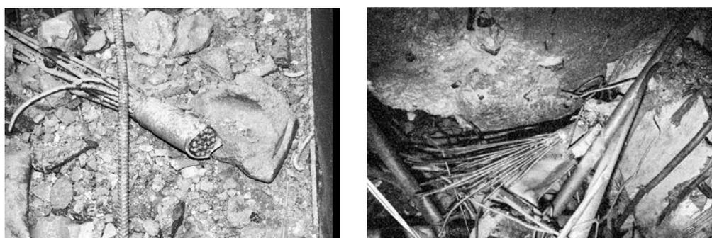
Fig. 3 Damaged fuel inside internal premises of the destroyed Unit 4
