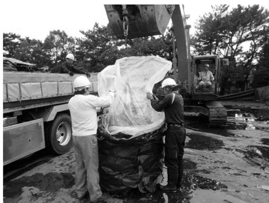
Fig. 4 Refilling contaminated soil
