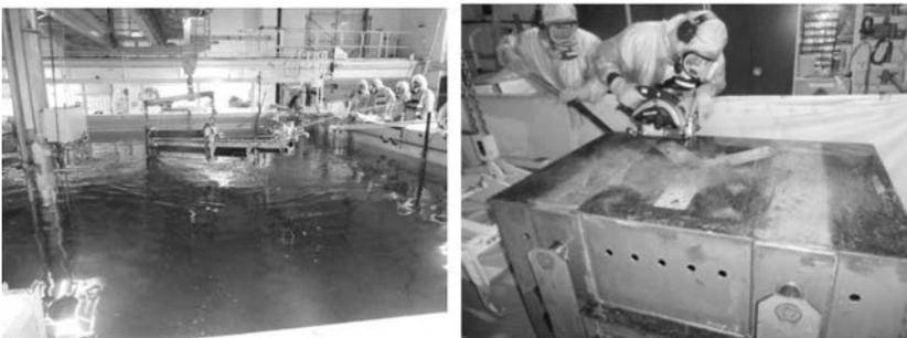
Fig. 13 Desplitter machine removal (left) and flat top size reduction (right)<sup>21)</sup>
